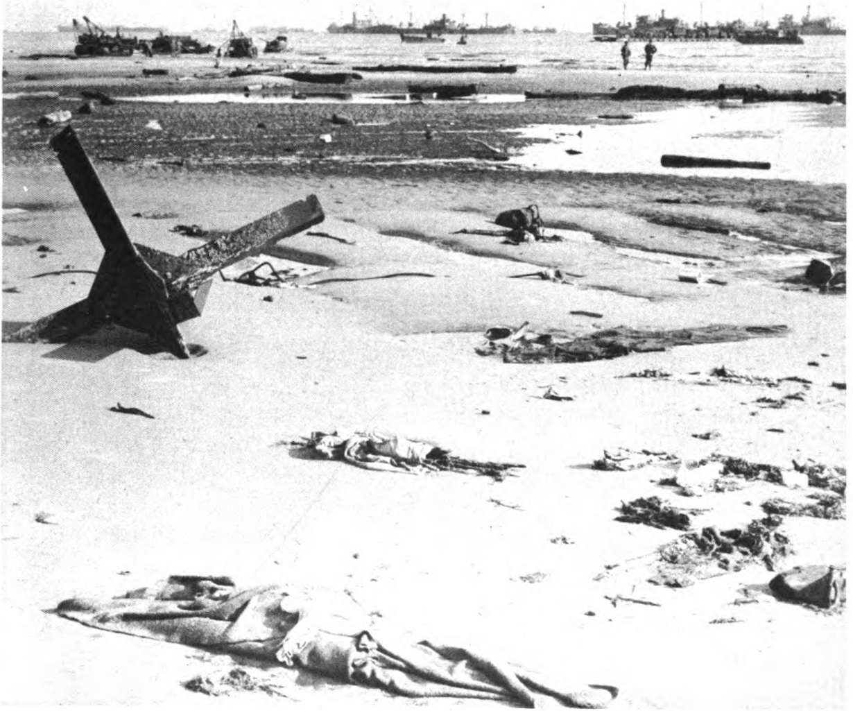
After— Land View of the Demolished Obstacles
